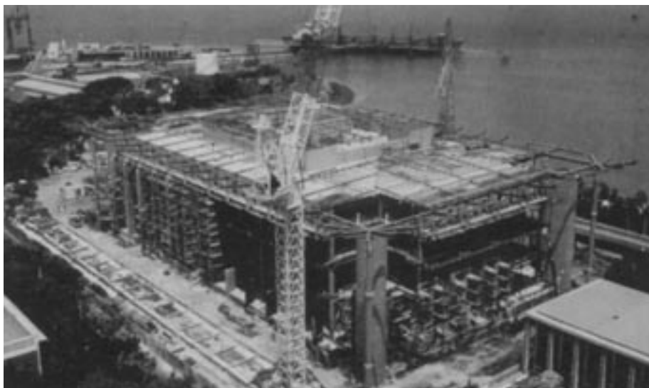
Photo 2: Northern Territory Parliament House – extensive use was made of AS 3597 grade 600 in the columns and transfer beams due to predicted cyclonic wind loadings
