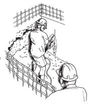
Further (as noted above), for concrete cutting or drilling, the operation of an internal combustion engined machine may produce additional extremely toxic gases in the confined space.
